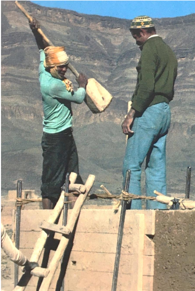
Traditional Rammed Earth Construction | Detier (1981)
